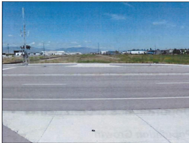
Locust Road crossing
